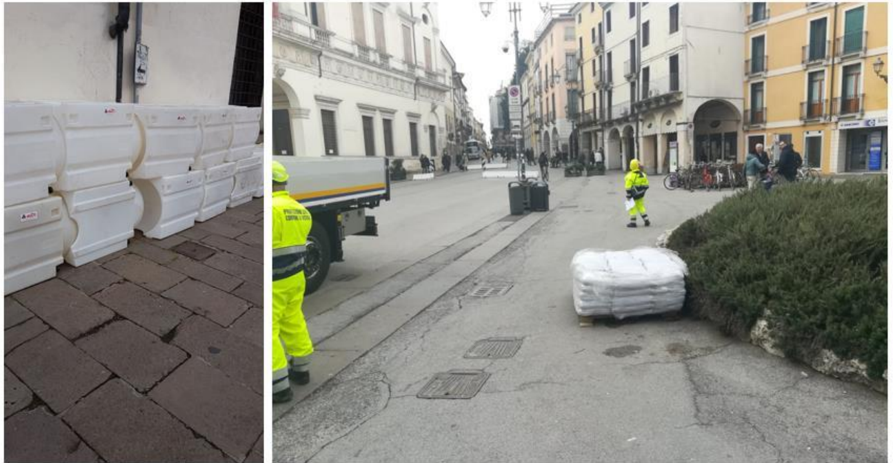
Figure 13. On the left: Aquadike placed during the pilot; on the right example of sand packs placed by the team
